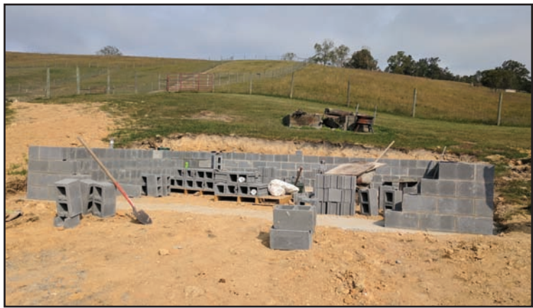
Space being constructed for the barn.
